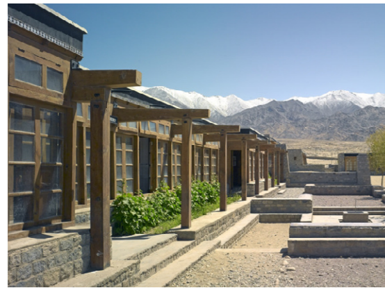
Figure 6.30: Exterior view of the Druk white Lotus School. ( https://www.dwls.org/sustainability/buildings-photo-gallery.html#prettyPhoto )
