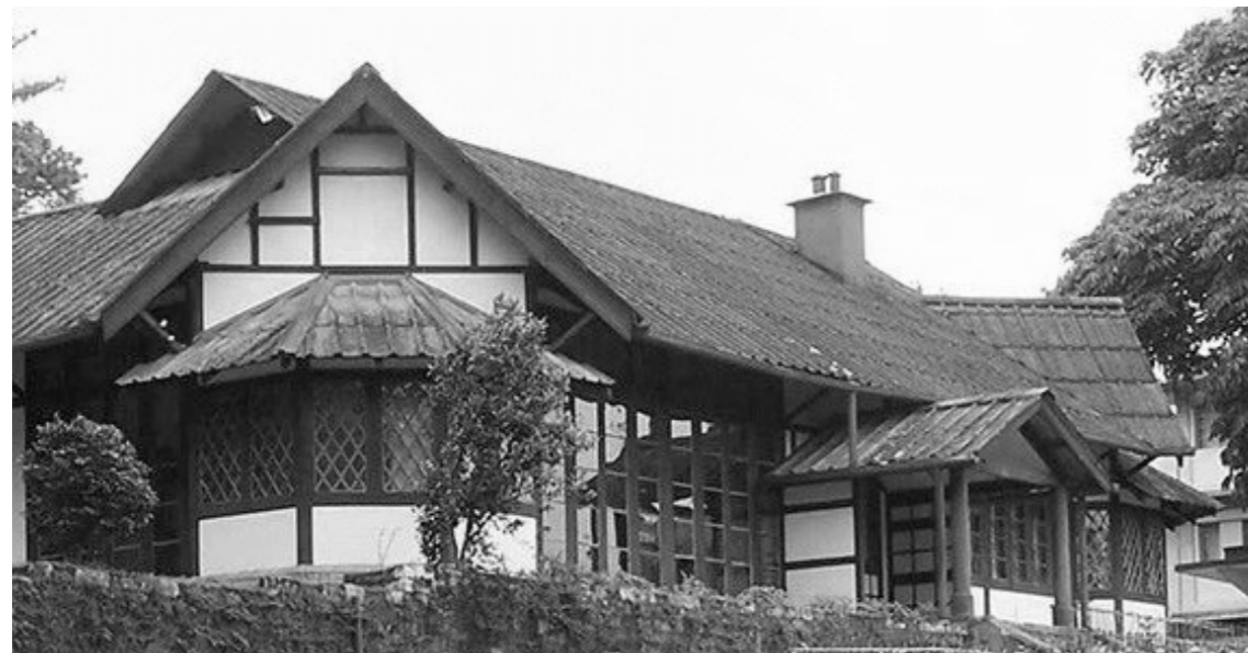
Figure 1.7: Image of an Assam type construction in Shillong.
