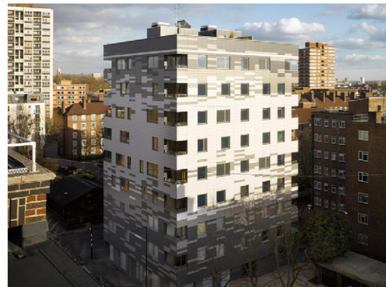
Figure 6.19: Exterior view of the Stadhaus. ( http://waughthistleton.com/murray-grove/ )
