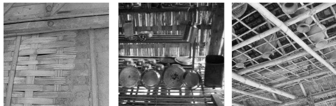
Figure 4.12: Left: Bamboo mat wall with mud plaster, Middle – Interior of a stilted house showing permeable floor, Right – Interior showing a bamboo loft. The above images are examples of bamboo uses in neighboring areas. [Source: (Nag & Gondane)].
