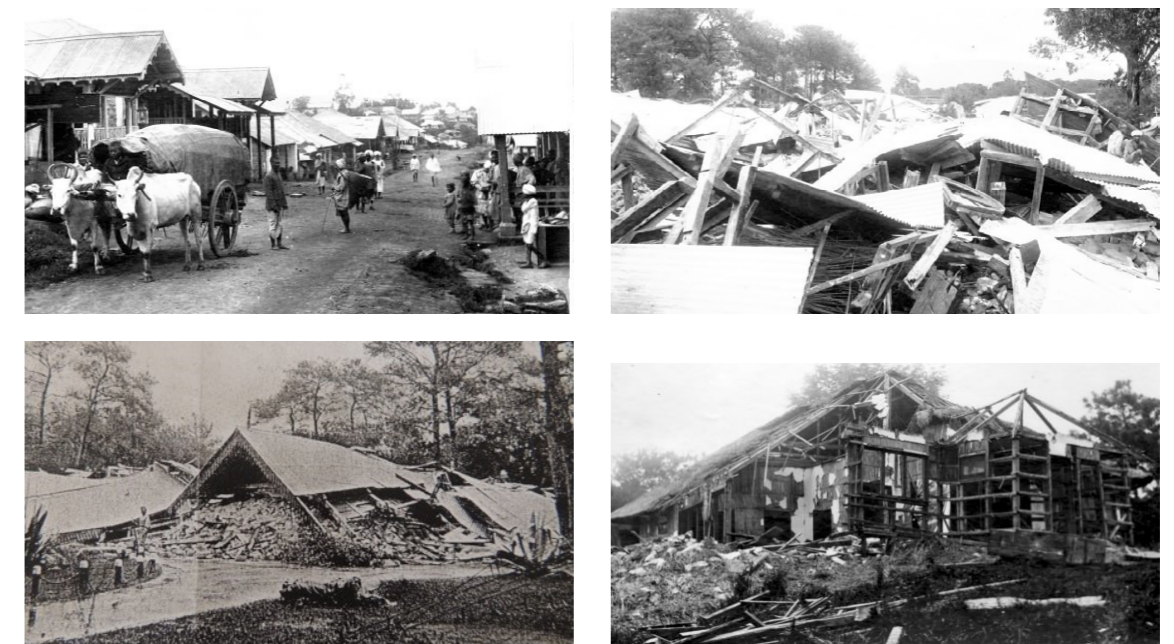
Figure 1.6: a) The Shillong market before and b) after the earthquake; c) ruins of governors house d) ruins of a cottage owned by a British. (Image source: https://www.seismosoc.org/Publications/SRL/SRL_79/srl_79-3_hs_esupp/ ).
