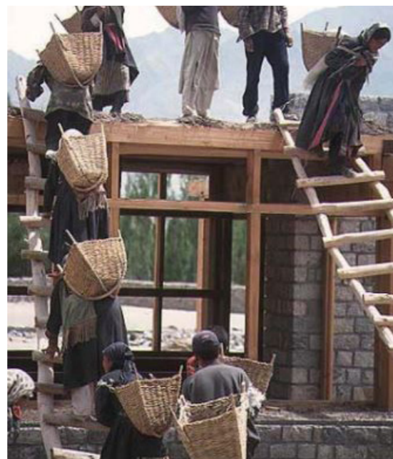
Figure 6.34: Construction progress. ( https://images.adsttc.com/media/images/5304/25f8/e8e4/4ee8/ac00/00b6/large_jpg/D1.jpg?1392780753 )
