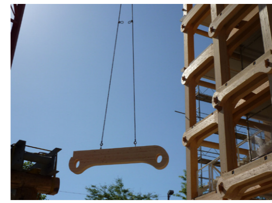
Figure 6.28: Construction progress. ( https://images.adsttc.com/media/images/5304/25f8/e8e4/4ee8/ac00/00b6/large_jpg/D1.jpg?1392780753 )
