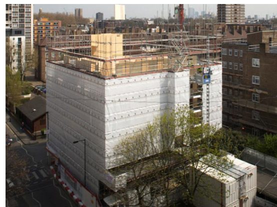
Figure 6.23: Construction progress. ( http://www.klhuk.com/portfolio/residential/stadhaus,-murray-grove.aspx )
