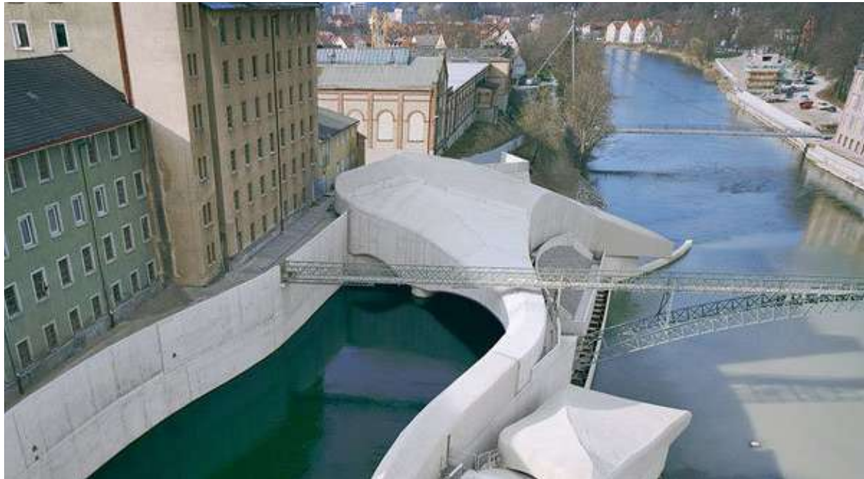
Hydroelectric Powerstation by Becker Architects, Kempton Germany
