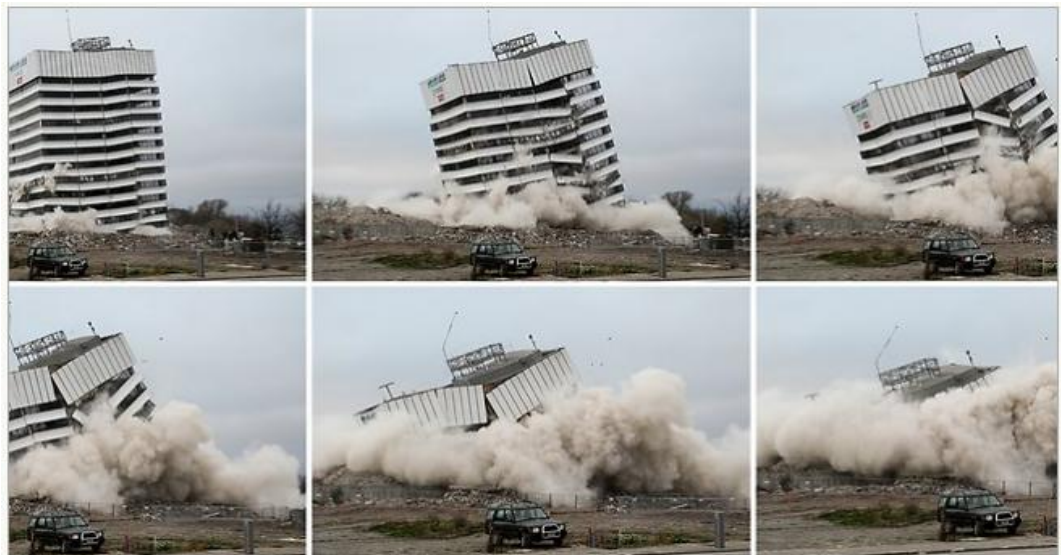
Figure 2.25 – Implosion with controlled explosions of a 14-storey building in New Zealand [Source: www.heraldsun.com.au/news/cancer-patient-jayden-halliwell-helps-implode-quake-damaged-building-in-christchurch/story-e6frf7jo-1226443136766]
