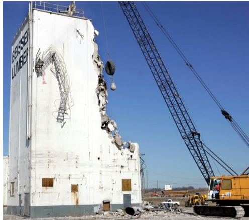
Figure 2.23 – Demolition of a building with wrecking ball [Source: archiveattic.wordpress.com]
