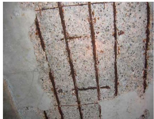
Figure 3.29 - Delamination / spalling
