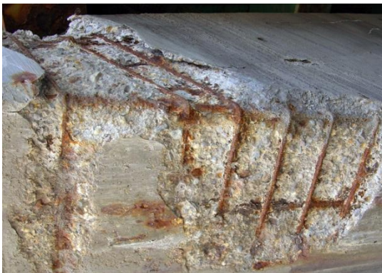
Figure 3.26 - Corrosion
