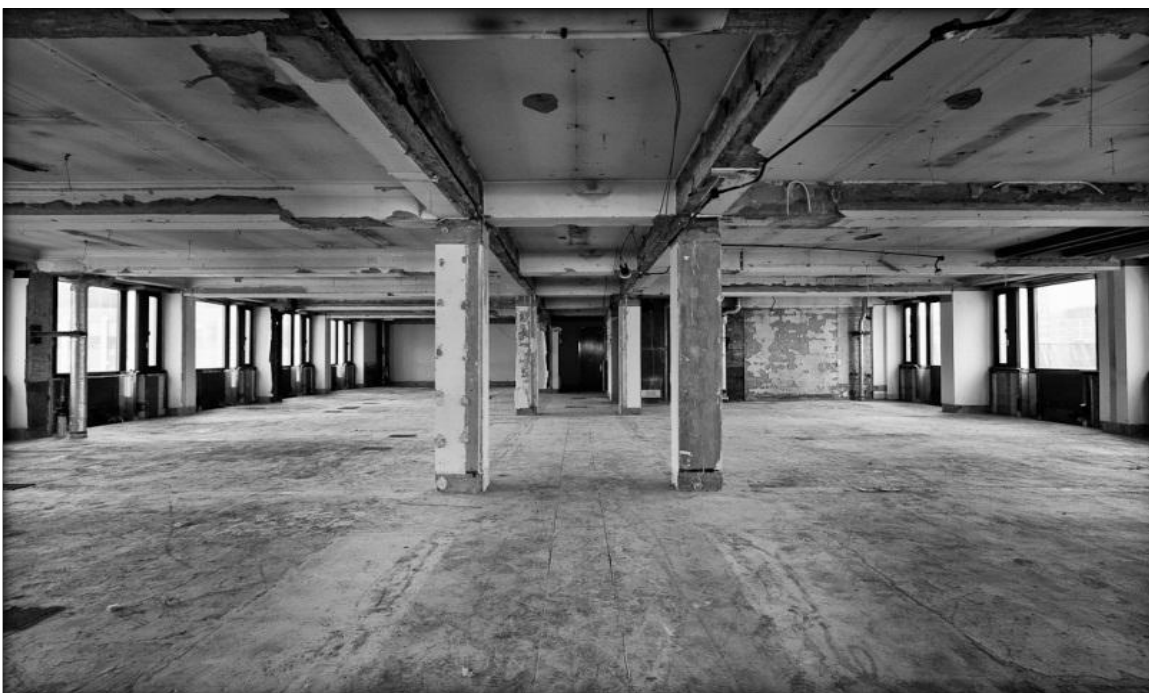
Figure 3.17 – Building stripped from inside (Source: www.ggardner.myzen.co.uk/wordpressblog/?p=2250 )
