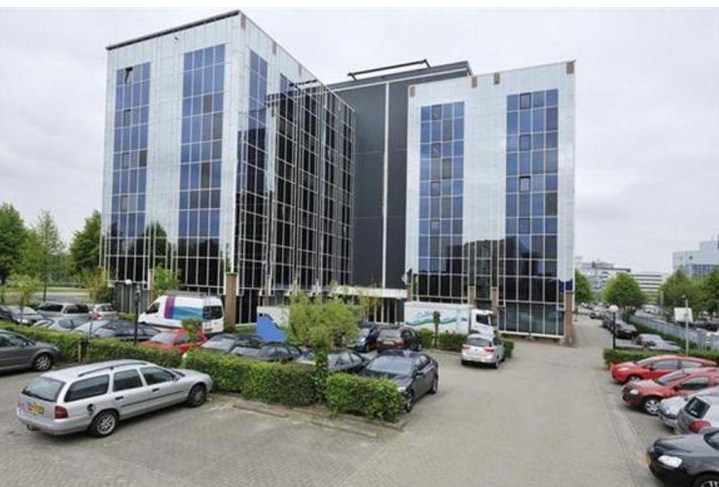
Figure 3.11- Office building on Karspeldreef 2
