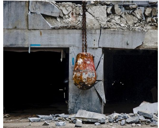
Figure 2.24 – A wrecking ball hits a column [Source: www.relocationfocus.com/]
