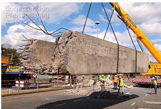
Figure 2.28 – Lifting of a section of a footbridge [Source: www.gilldemolitions.co.uk ]
