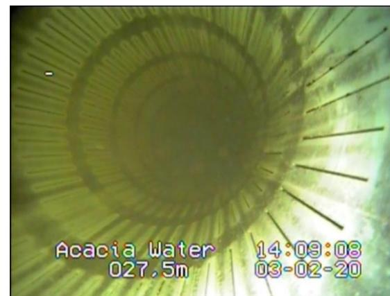
Figure 3.14b: In-well condition after the well rehabilitation. Horizon is the exact same as 3.13b.
