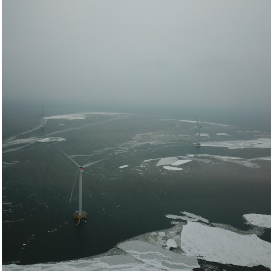
(a) Offshore wind turbines in icing conditions at the Nissum Bredning Vind Offshore Wind Farm in winter of 2018 (Siemens Gamesa Renewable Energy, 2018).
