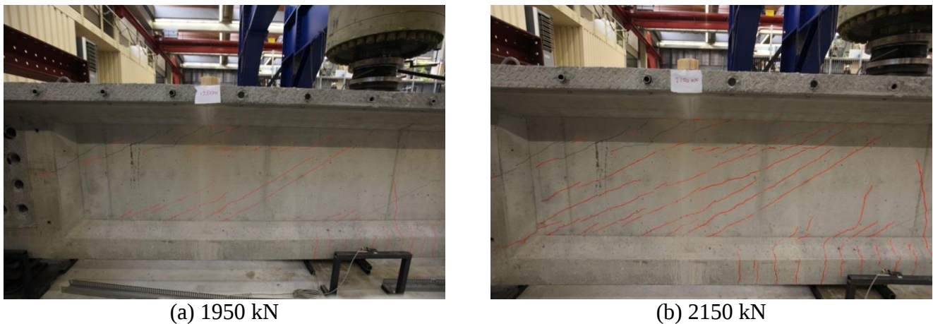
Fig. 9 Crack development beam type 101 (first test)
