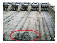
Figure 1.2: Pitting erosion-wear effects of cavitation due to the violent cloud collapse: (a) ship propeller (Asnaghi, 2015), (b) throttle valve (taken from tameson.com, the image is made available by Scott Louis Simonson), (c) pump impeller (Pokharel et al., 2022), (d) dam-spillway erosion encircled in red (Mittapalli, 2015).
