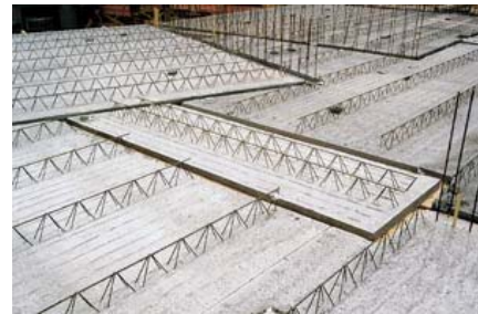
Fig 4-12 Composite plank floor (Dycore)
