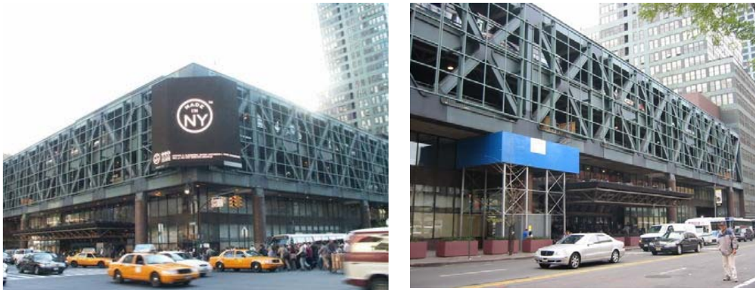
Fig 7-4 Port Authority Bus Terminal, USA
