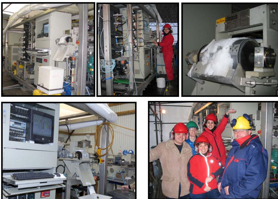
Figure A2: Demonstration of EFC Skid at AVR Industries, Rozenburg-Netherlands, March 2007
