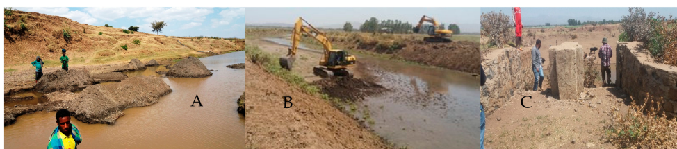
Figure 8. (A) excavated sand accumulation by sand miners in the Middle River reach; (B) river channel enlargement and deepening to increase flow conveyance. The contractor used the material for embankment construction at the Lower reach; (C) flood outlet structure to the farmlands as low height weir (April 2016).
