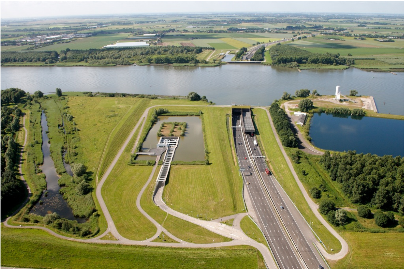
Figure 12: 2nd Heinenoordtunnel (left) and Heinenoordtunnel (right) [22]
