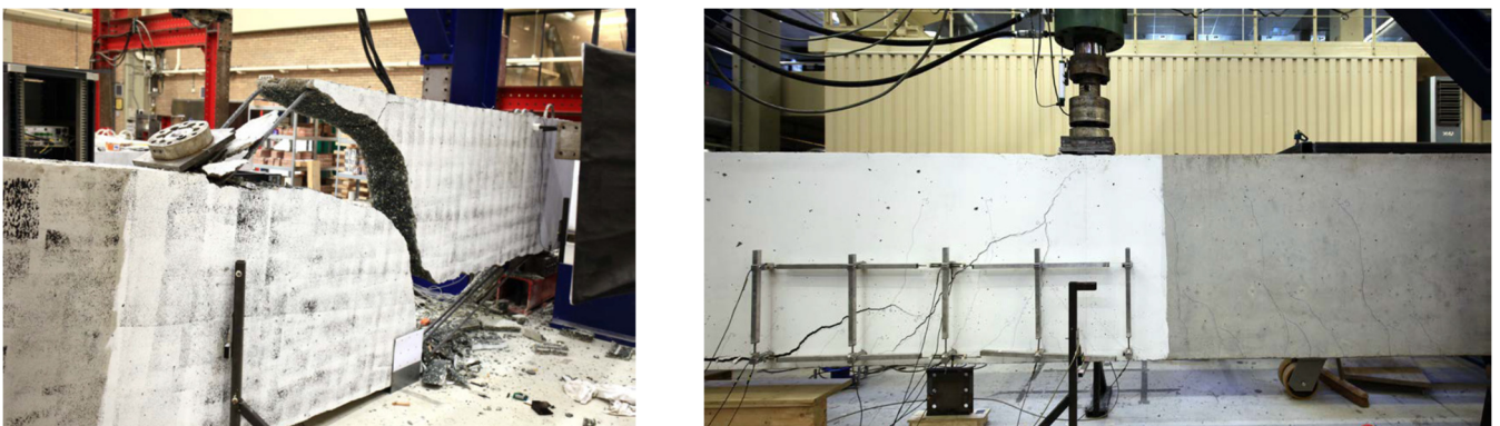
Figure 39: Spalling on concrete on test specimen H351 (left) and failure on test specimen H352 (right)
