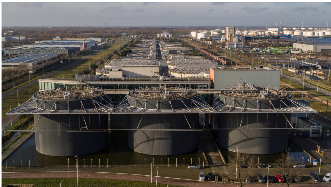
Fig. 4. Amsterdam West WWTP (Source: Waternet).
