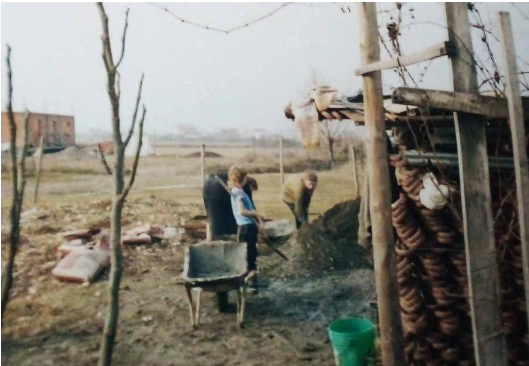
FIG. 6.18 Picture of mother and her children mixing concrete to construct their house, Source: Family archive
