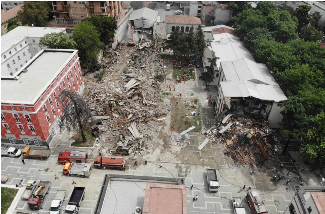
FIG. 7.5 Bird's-eye view picture taken during the early hours of May 17, 2020. The demolition started at 4:30. Picture taken by drone. Source: Behaudin Dobi
