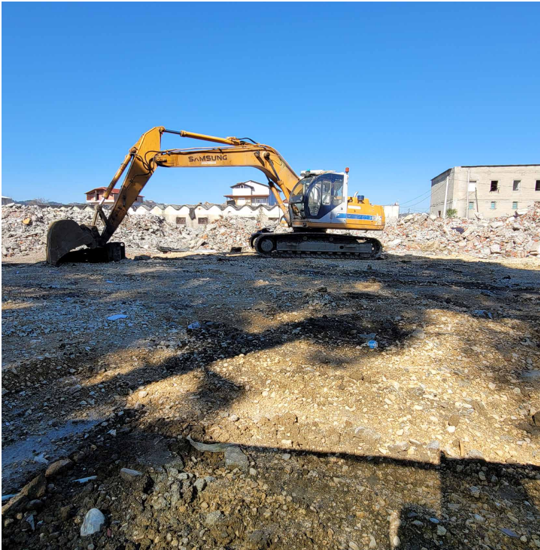
FIG. 5.1 Demolition of squatted former industrial buildings at Kombinat to make way for new apartment blocks envisioned in the Kombi-Art masterplan. Site visit 23.02.2022
