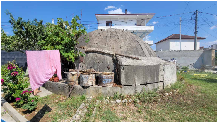
FIG. 6.14 The bunker is a solid presence in the yard
