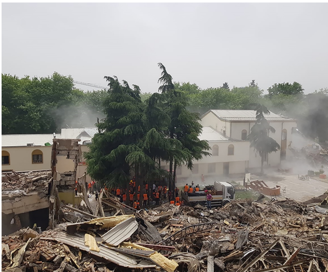
FIG. 7.12 Picture taken by drone during the early morning hours of May 17, 2020. Source: Edmond Dingu
