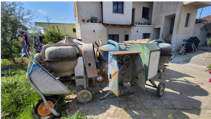
FIG. 6.15 Construction machinery in the yard indicated that the construction work continues
