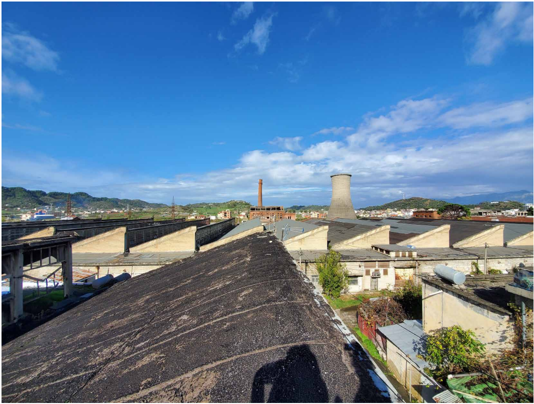
FIG. 5.16 Photo taken from the rooftop of Hidrofilii looking toward the former Factory of Thin Fabrics
