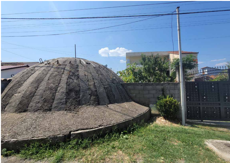
FIG. 6.13 The bunker is made part of the external wall of the parcel.
