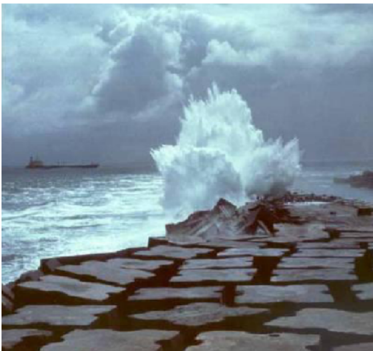
Figure 1.1: Sines (Portugal) breakwater under wave attack
