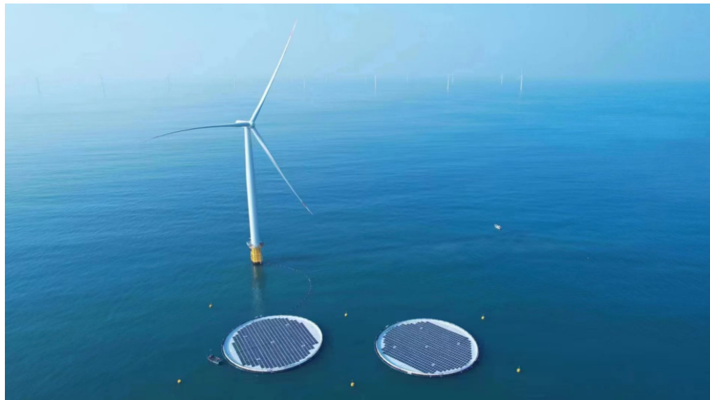
Figure 2.9: First off-shore solar farm (0.5MWp) integrated with an off-shore wind turbine (Santos, 2022).
