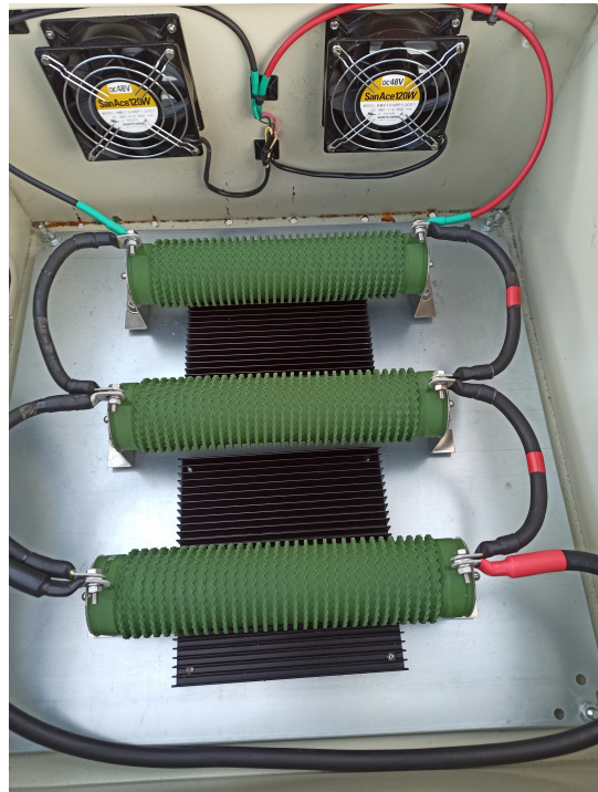
(b) Resistors box components installed.
