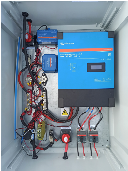
(a) Power box components installed.
