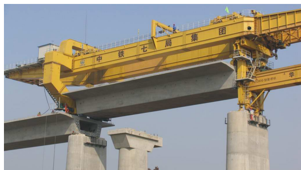
Fig. 27 - Span by span construction method [22]
