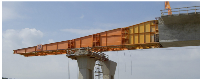
Fig. 29 - Incremental launching method [24]
