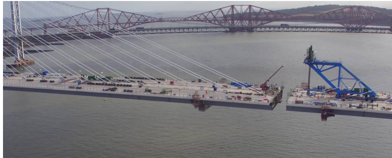
Fig. 28 - Balanced cantilever construction method [23]
