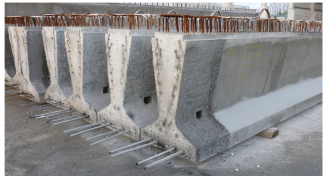
Fig. 10 - Prestressed precast concrete beams [9]
