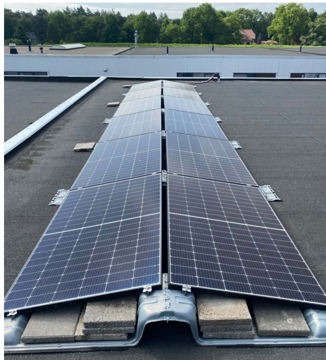
Figure 4.6: PV solar panels used for the experimental setup. The setup features 12 PV solar panels, connected in parallel. The panels are divided into two 6-panel groups. One group is East-facing and one group is West-facing.
