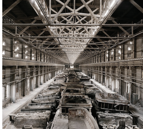
Figure 3.3: Dilapidated factory with reusable steel truss and interior space (photo by Edward Burtynsky)
