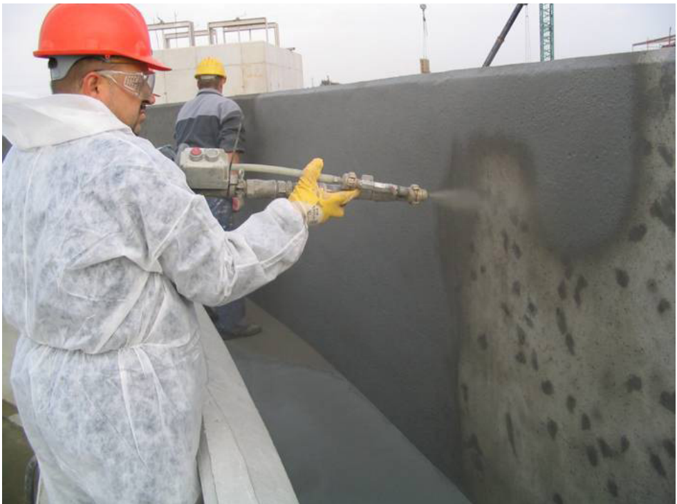
application of spray concrete
