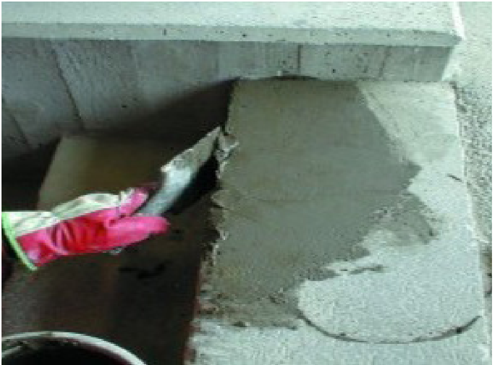
application of repair mortar
