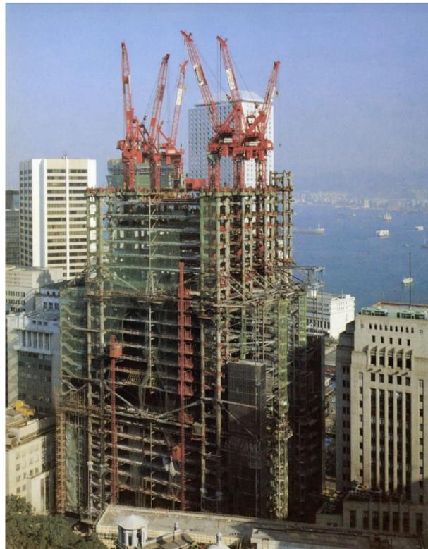
**Figure 5:** Photo of the construction of HSBC Building. From Avery/GSAPP Architectural Plans and Sections (Columbia University). 1979. Source: Foster Associates.
