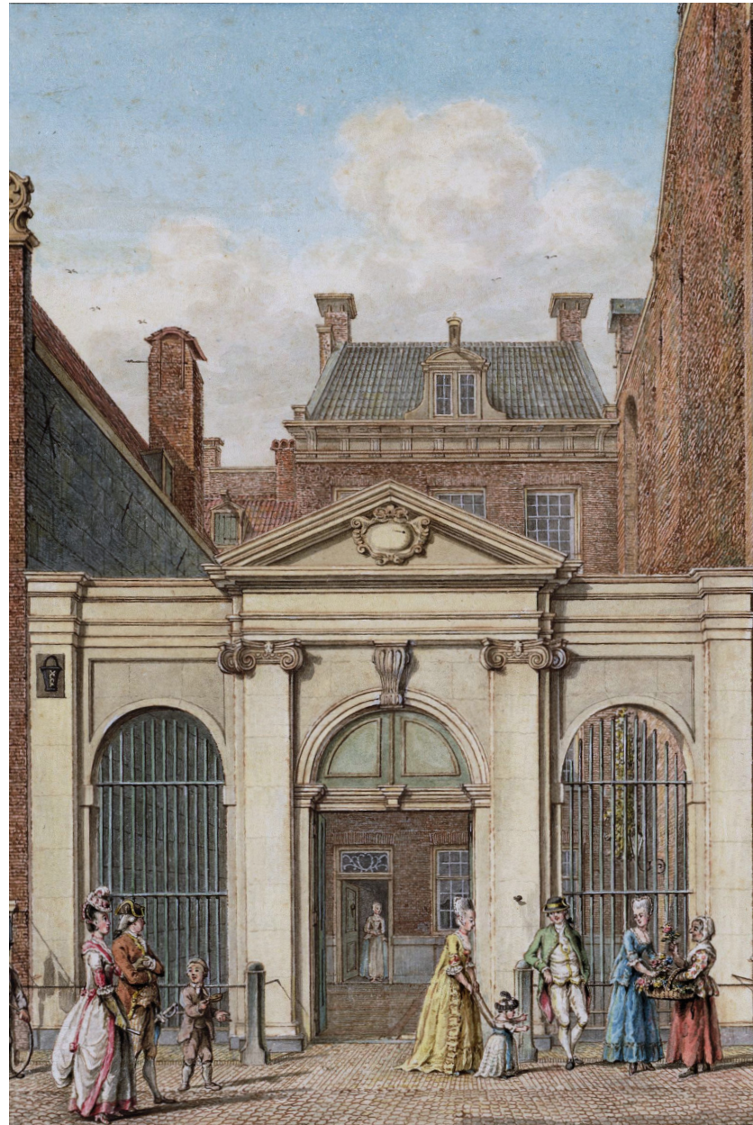
fig. 08: entrance theater van van campen historic painting
