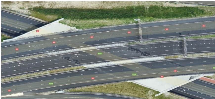
Figure 1.1: A skewed slab highway bridge in the Netherlands, where additional triangular segments were applied, from [3]
