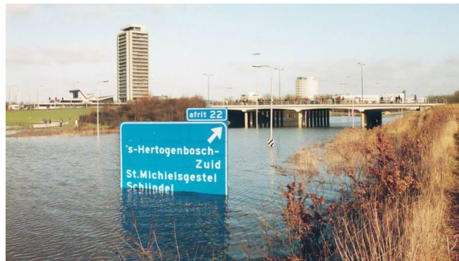
Figure 3.2: Flooded A2 as a result of a dike breach of the Dommel river in 1995 (Brabants Historisch Informatie Centrum, 1995)
