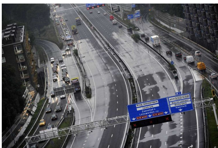
Figure 1.2: Local flooding of the A10 highway after a precipitation event of 40 mm in one hour in July 2014 (Volkskrant, 2014).
