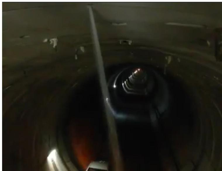
Figure 1.2: Water gushing into the tunnel in the Middle-East case
