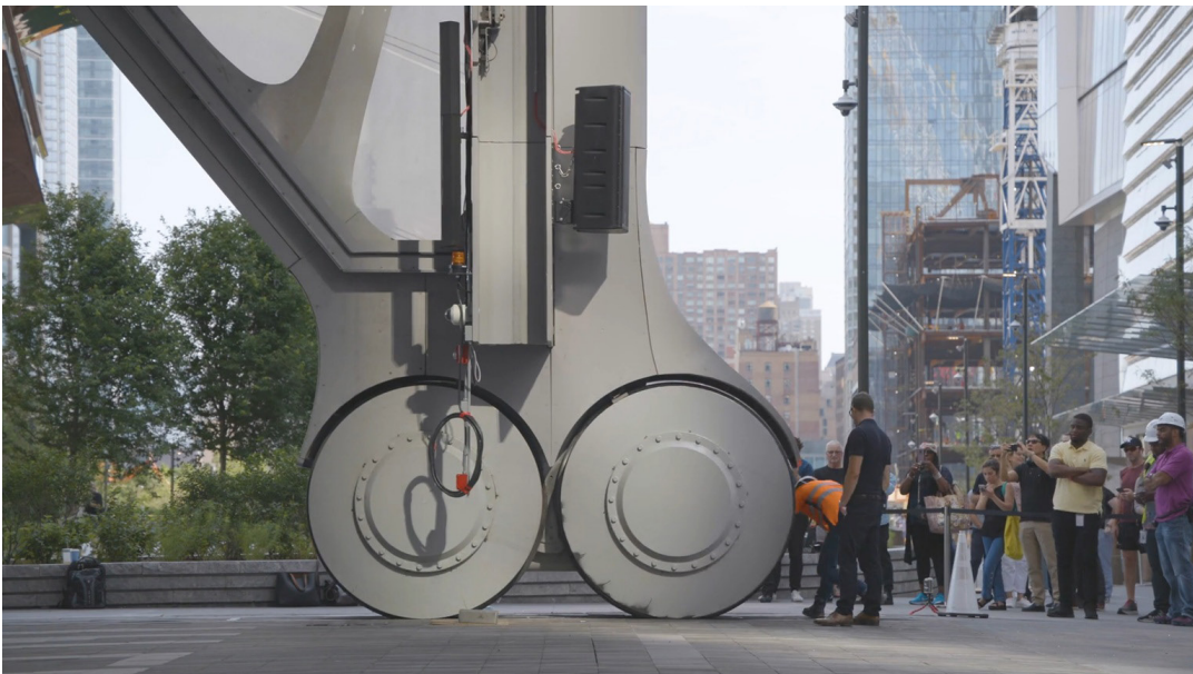
Figure 45. Video capture of the testing of the movable shell of The Shed , showing the wheel mechanism that enables large-scale transformation.
