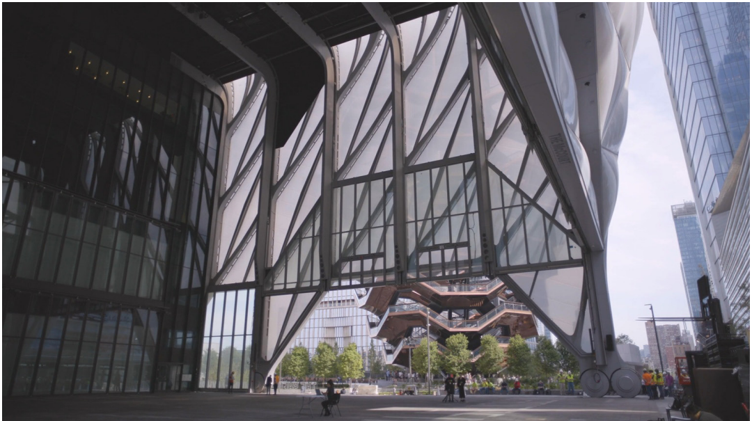
Figure 44. Video capture of The Shed , showing the movable outer shell deploying over the plaza.
