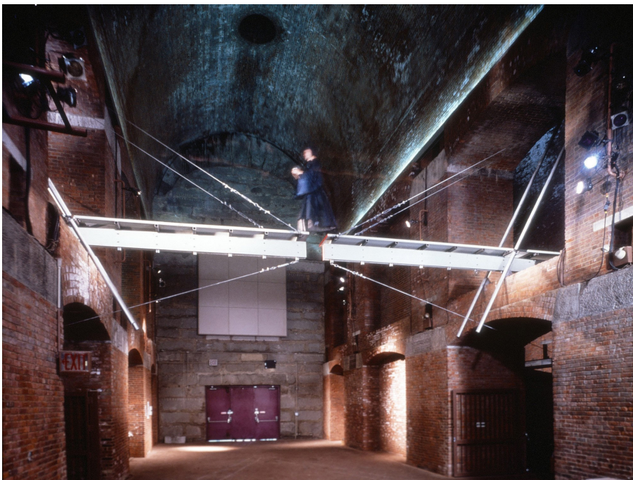
Figure 34. Photograph of Camillo's Bridge , showing its minimal structural supports.
