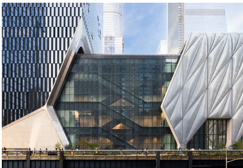
Figures 17–18. A large wheel during the construction of The Shed (2019) and the completed project, illustrating the wheel mechanism that enables the building to physically transform for different events.
