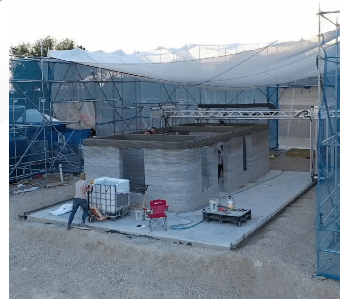
Construction site ICON with their Vulcan 3D printer
