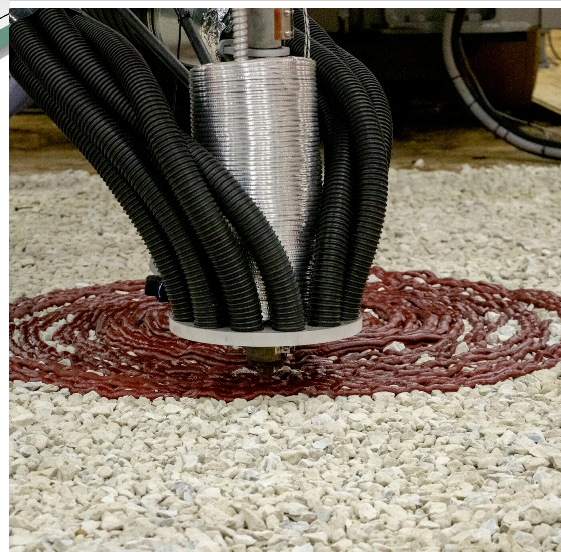
Foundation beams printed on earth like AI Spacefactory
