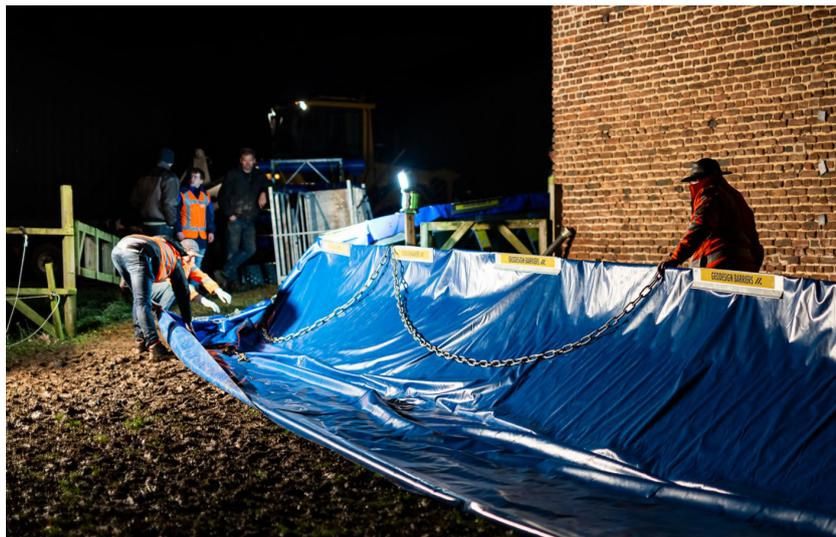
**Figure 1.2:** Installation of the Geodesign Barrier on December 22, 2023, as reported by Waterschap Limburg
