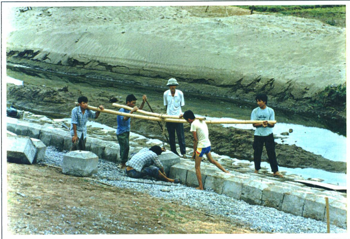
Photo 12 Construction of new protection on second dyke, Hai Thrieu
