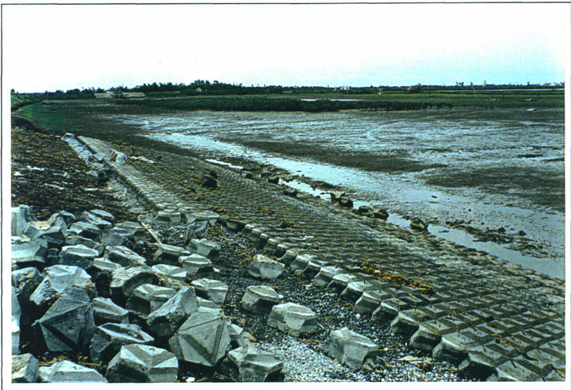
Photo 4 Construction of slope protection on single dyke, mangroves
