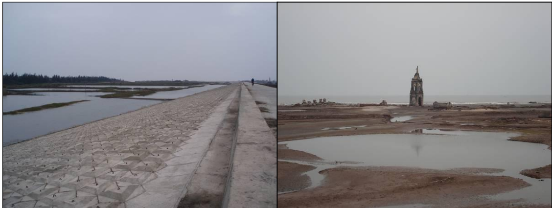
Figure 21: Second dike has become first dike (left) and erosion in Hai Hau district [photo: Hillen (left), photo: Huong (right)]
