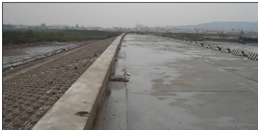
Figure 16: Restored sea dike Hai Phong province, left is sea-side [photo: Huong]
