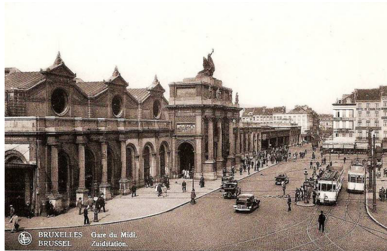
South station from 1869 by architect A. Payen. Photo: Skyscrapercity.com, 2010
