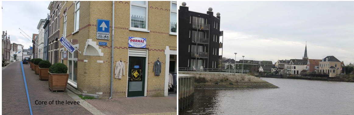
Figure 18 - Levee in Moordrecht (left), urban developments on the levee (right)
