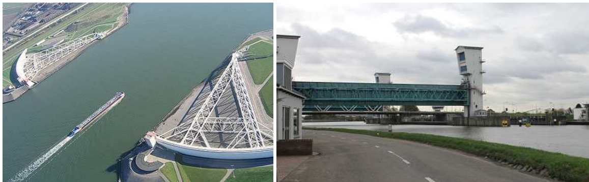
Figure 12 - Maeslant (left) and Hollandsche IJssel (right) storm surge barrier, source; omroepwest
