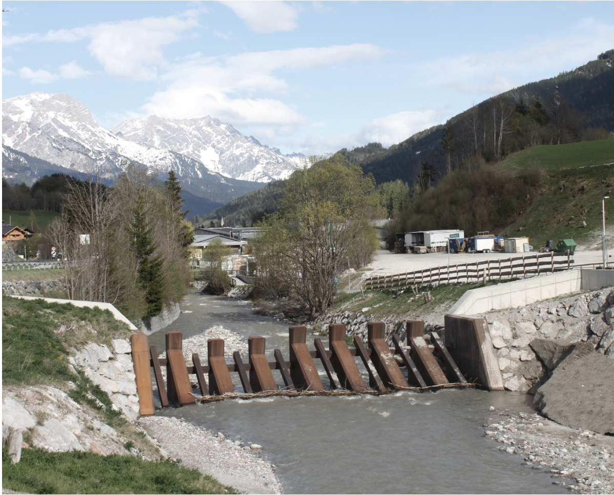
Figure 44: Barrier structure in the torrent 'Leoganger Ache' Source: Author
