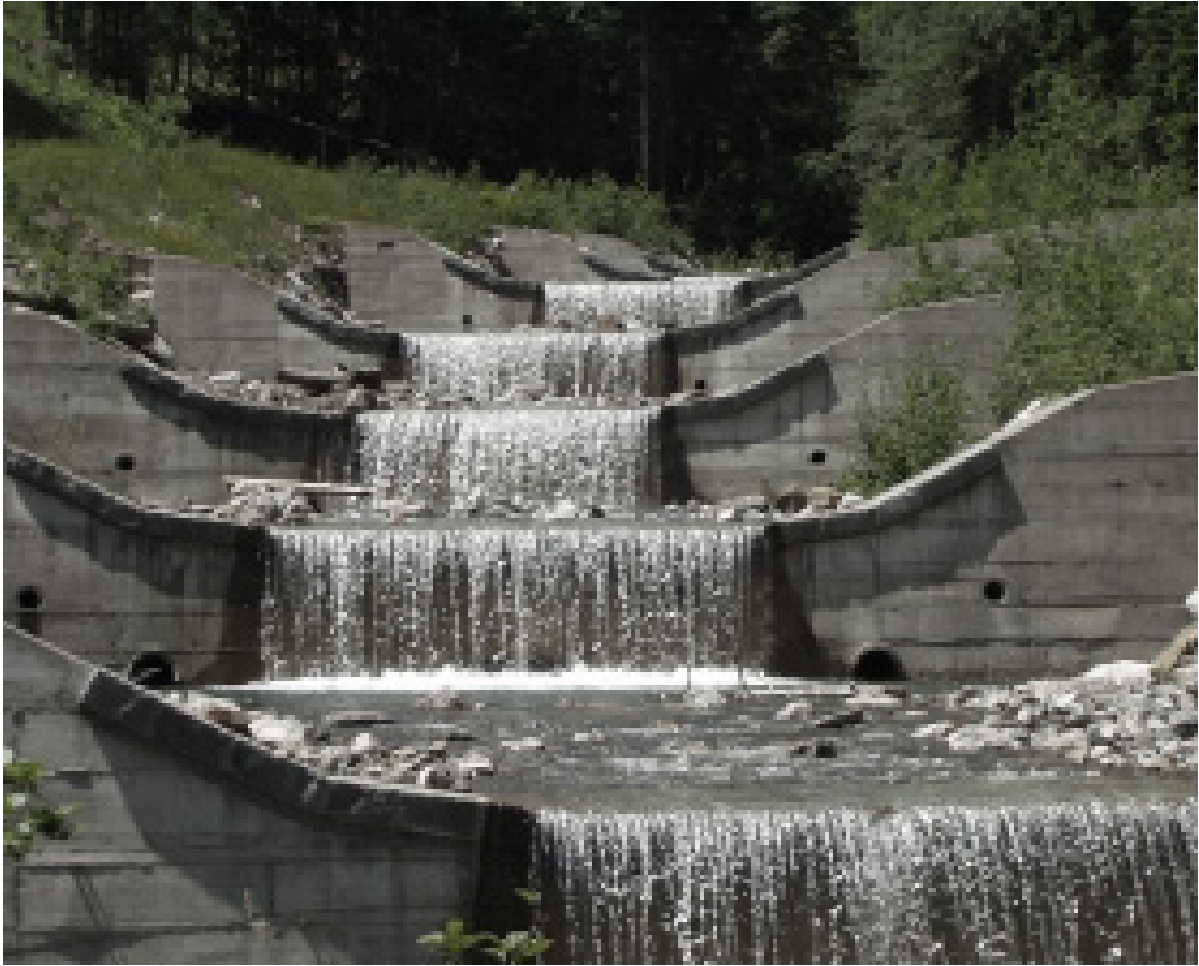
Figure 45: Drop structure in torrent Source: www.biberberti.at
