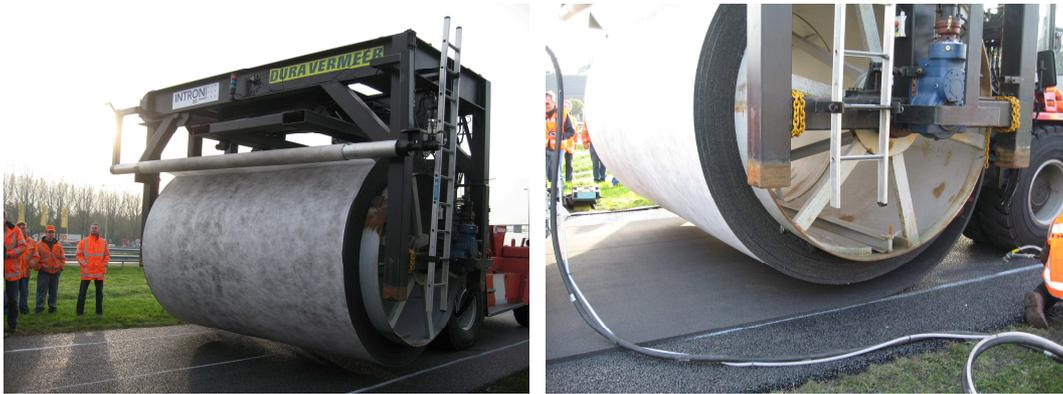
**Figure 2-7 Transportation and laying of the Roll Pave**
