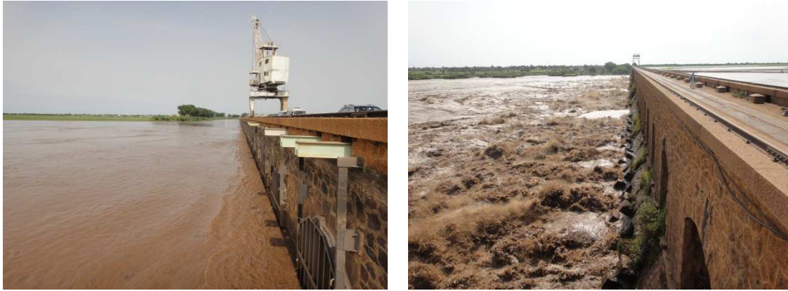
Figure 2.8: Sennar Dam during flood season, upstream (left) and downstream (right).
