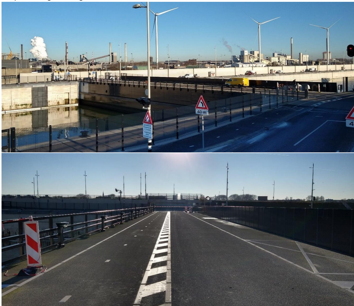
Figure 1.1: Lock door IJmuiden with retreated wall on the right (design wave enters from left to right). By H. G. Tuin, n.d.
