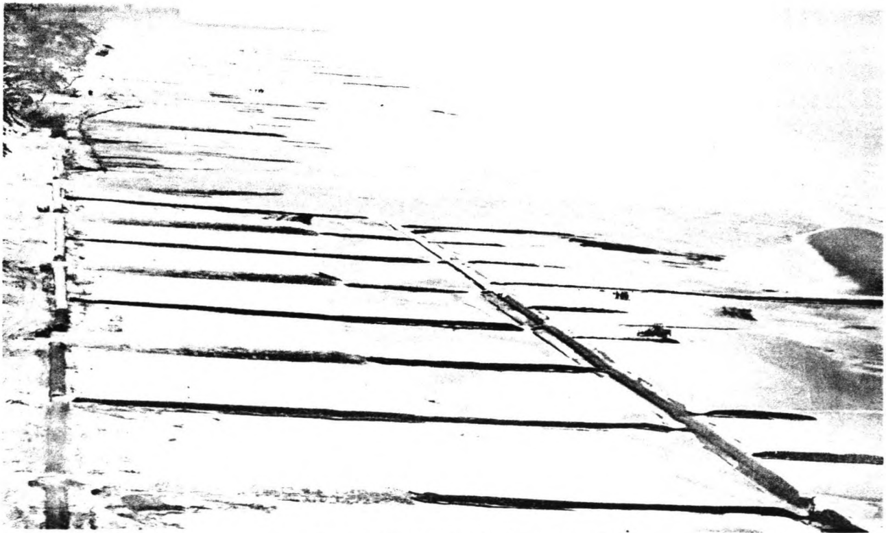
Coast protection project from Klemskerke, Belgium.
