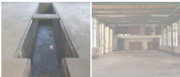
fig. 9 - Inspection pit and checker flag tile detail (own images, 2016)
