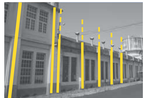
fig. 10 - extension of car-workshop
