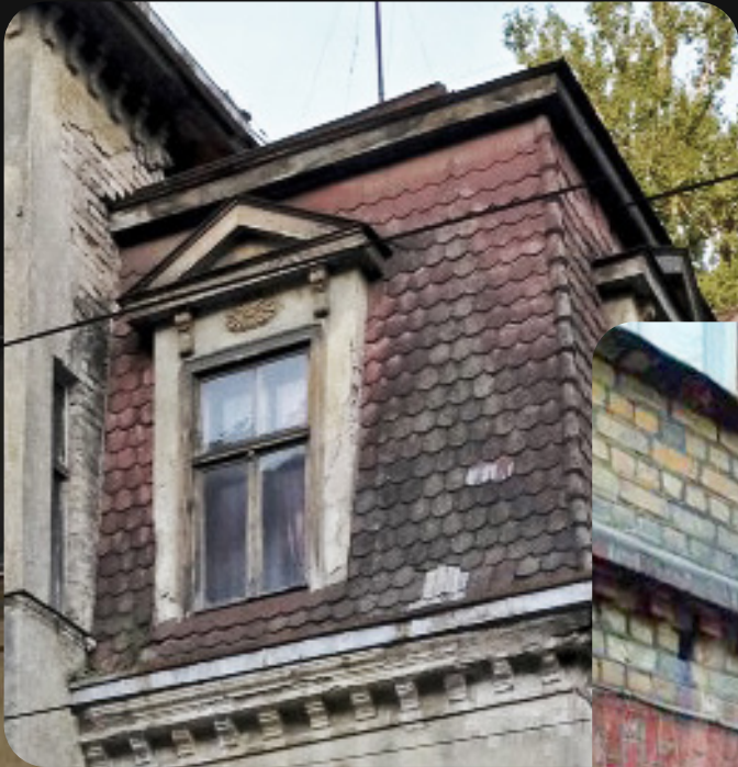
Rounded roof shingles
