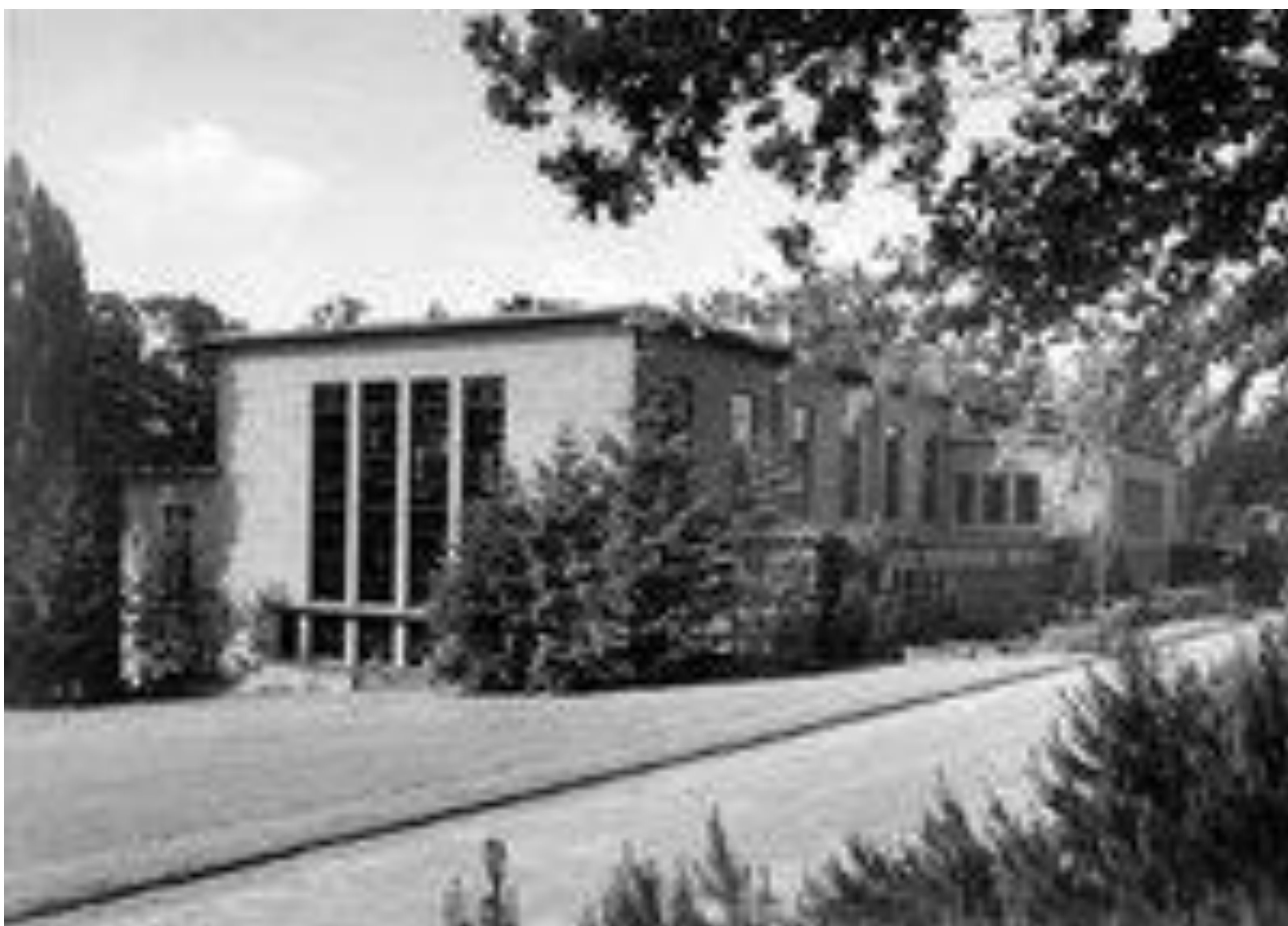
Figure 3. High voltage Laboratory designed by H. Fels and R.A.L. Schoemaker in 1937
