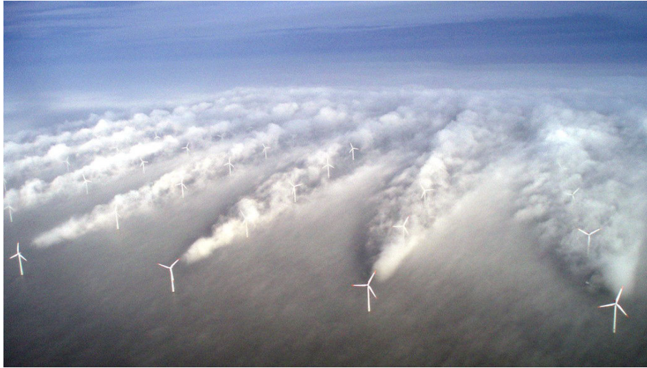
Figure 1-1: A depiction of wind turbine wakes in a wind farm. Source: Christian Steiness.
