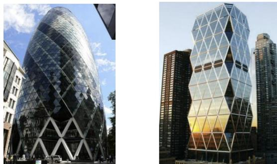
Figure 86. Diagrid structures. (a) Swiss Re[47] (b) Hearst Tower[48]
