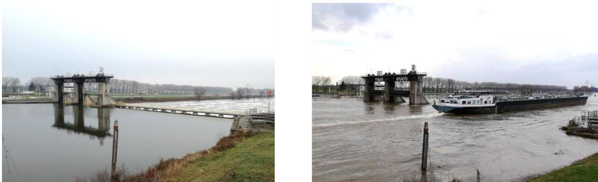
Figure 2-10: Photographs of weir Belfeld in a dammed river mode (left) and a free flowing river mode (right).
