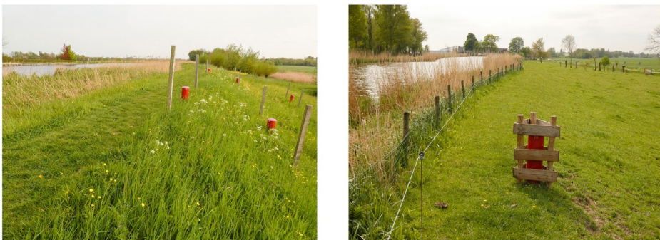
Figure 3.1 Two examples of canal dikes in the Netherlands: Duifpolder is shown on the left and the Drooggemaakte Geer- en Kleine Blankaardpolder is depicted on the right. In both images, the canal has permanent high water levels close to the crest level (on the left side) and the low-lying polder is mainly used for agriculture (on the right side). The head differences between the canal water levels and water levels in the polders are 2.7 m (Duifpolder) and 4.3 m (Drooggemaakte Geer- en Kleine Blankaardpolder). The red tubes protect the measuring equipment and the piezometers used to measure the hydraulic head. Photos by EURECO/Cyril Liebrand (2022).
