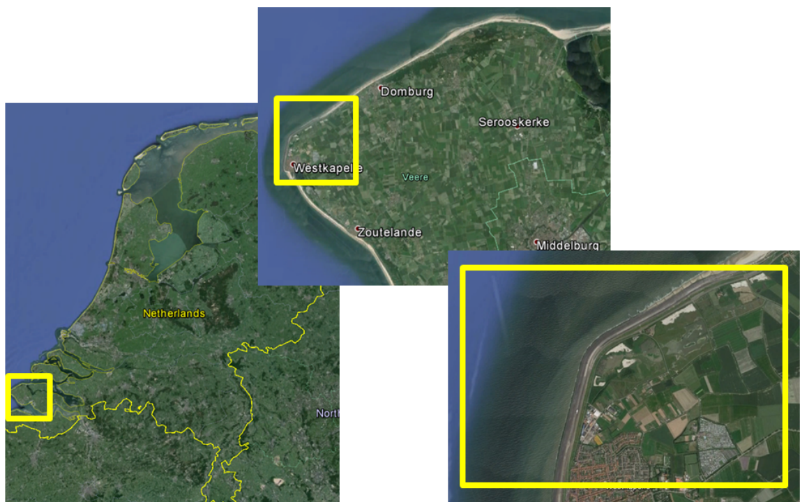
Figure 1.4: The Netherlands, the western part of Walcheren and the Westkapelle sea defence, running from the beach in the Northeast until the beach in the South. In this figure North is upward.
