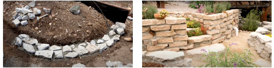
Figure 26 Retaining Wall ( https://www.youtube.com/watch?v=aM4FWHb75mE )
