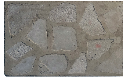
Large Stones Smooth Surface
