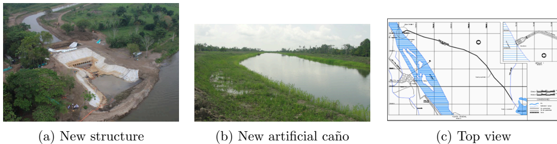
Figure 7.2: New hydraulic structure at Sogamoso river
