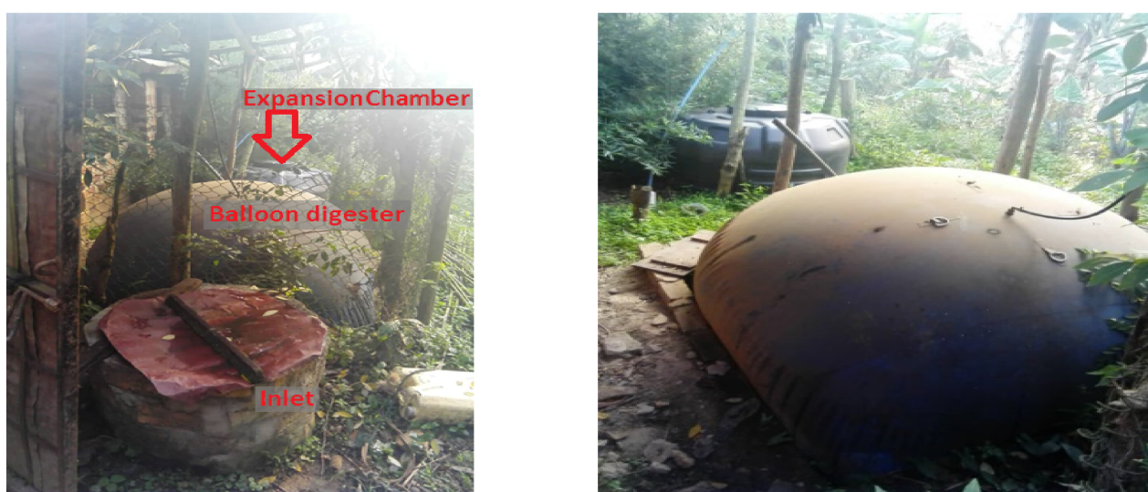
Figure 7. Balloon type digester.
