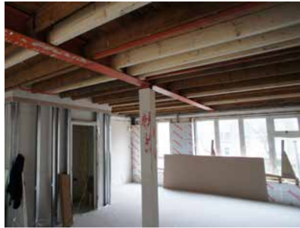
FIGURE 2 Koningvrouwen van Landlust, interior of a dwelling during renovation.
