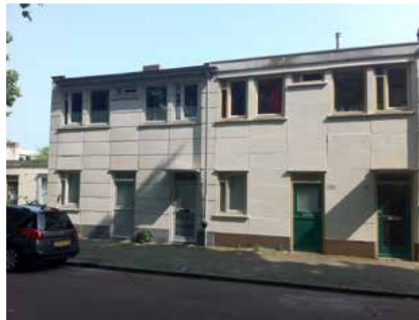
FIGURE 4 Jeruzalem. The pilot renovation project
