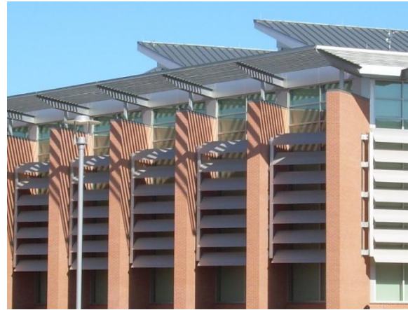
Figure 2.10 Useful for both shading & fire safety 15
