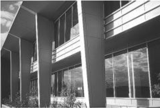
Figure 2.9 External projections as horizontal separation
