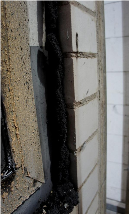
Figure 2.15 Intumescent sealant after Test 2
