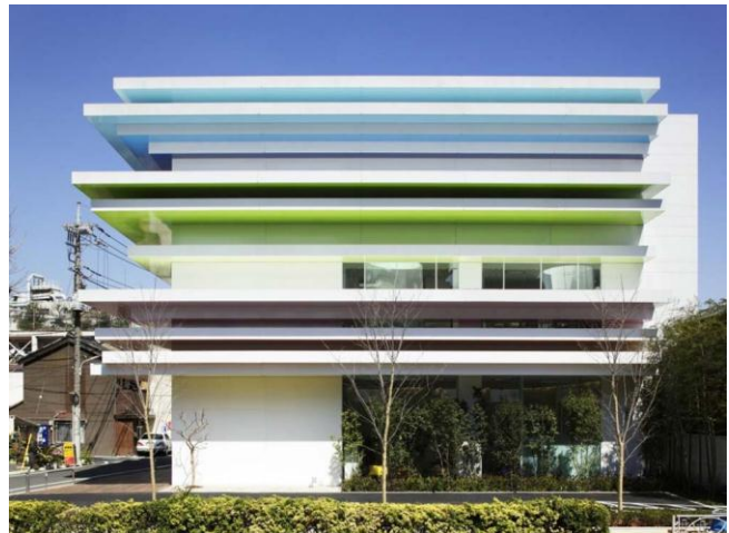
Figure 2.8 Façade with horizontal ledges 14
