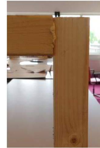
Figure 125: sealing the connections with silicone
