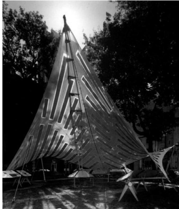
Figure 6: First photovoltaic tensile structure at the 'Under the Sun' exhibition at the Cooper-Hewitt National Design Museum, New York, 1998, designed by FTL Design Engineering Studio.
