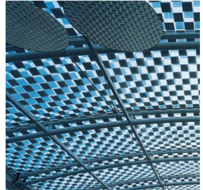
Figure 63: printed patterns on the ETFE membrane
