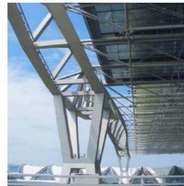
Figure 37: connection of the roof with the load-bearing structure
