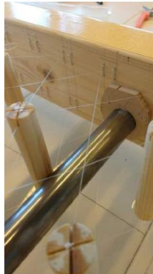
Figure 131: connection of the steel tube to the frame
